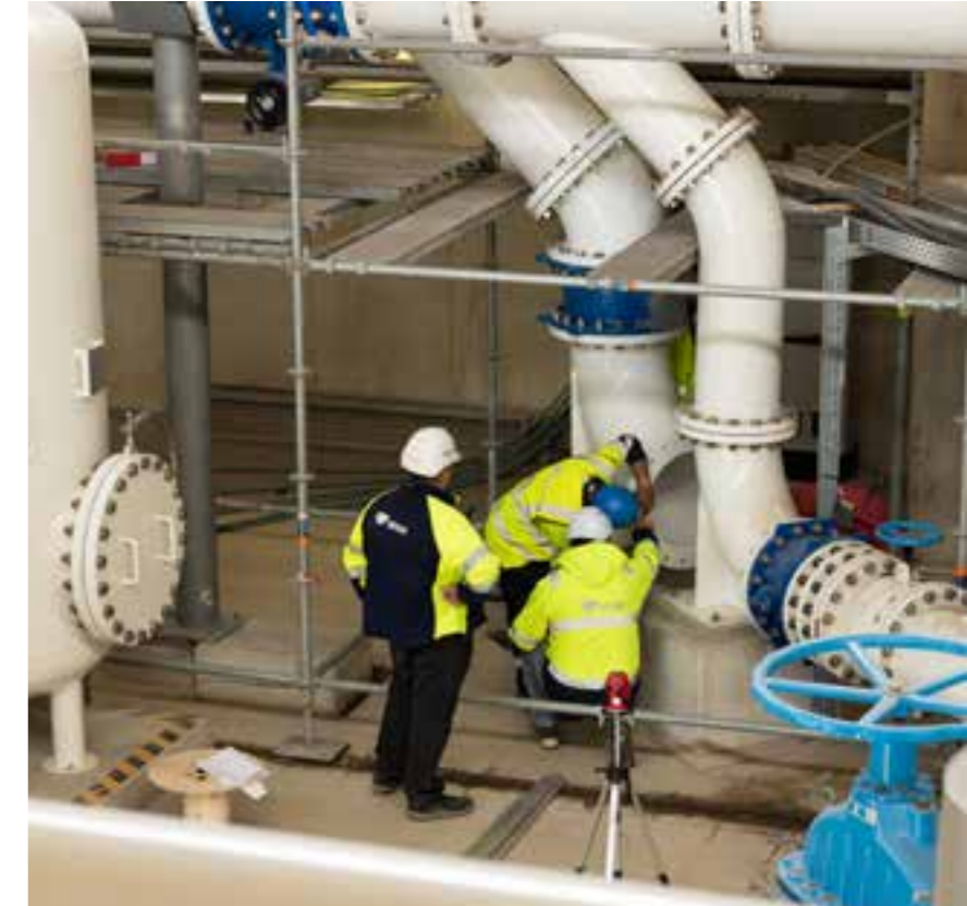
Renovation of the De Gavers water production centre in Harelbeke
