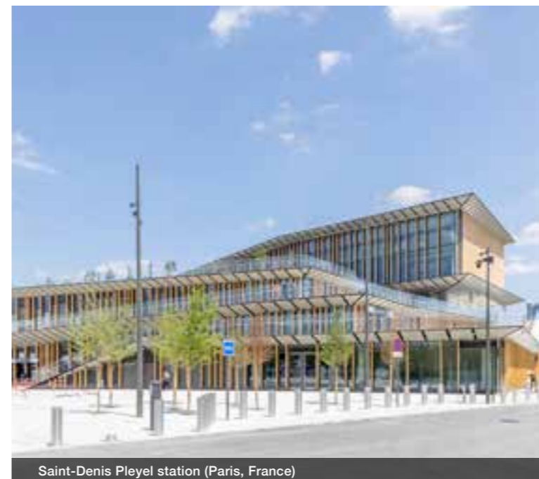
Saint-Denis Pleyel station (Paris, France)
