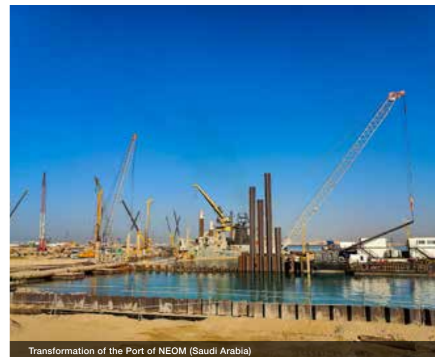
Transformation of the Port of NEOM (Saudi Arabia)
